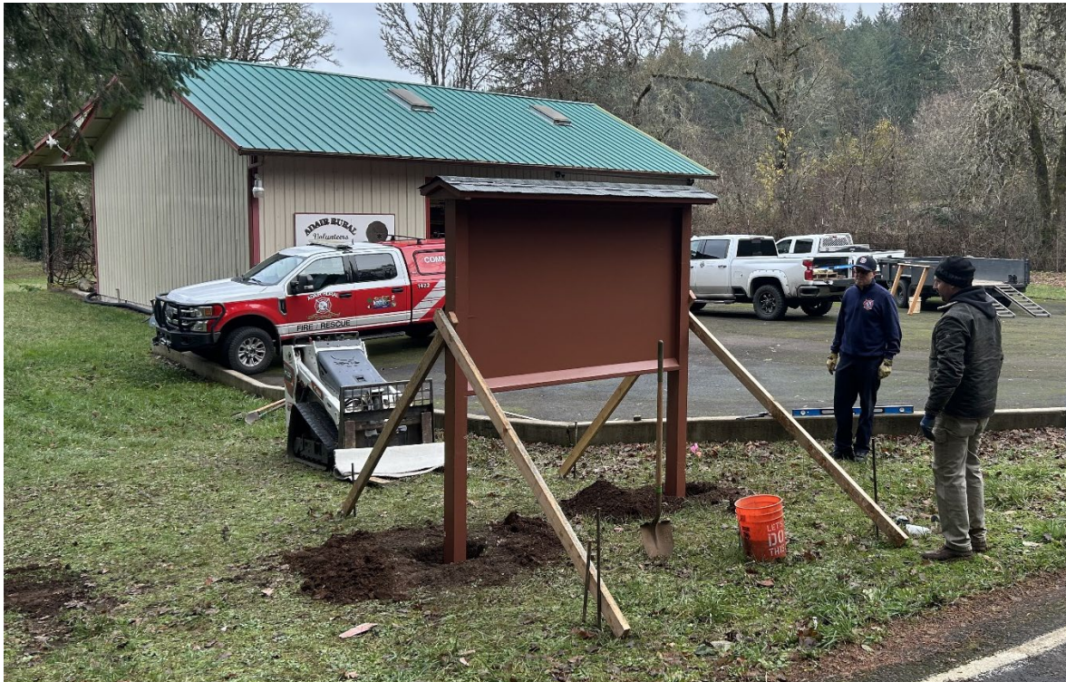
Installing the new sign at 1402.
